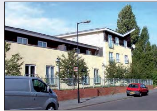
Lawrence Weston new flats
