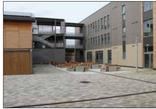
A sociable courtyard at Filwood Green
