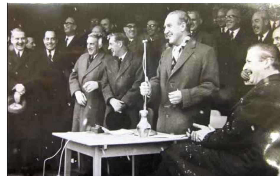
Transport Minister Ernest Marples at the opening ceremony of Phase I of the Cumberland Basin Bridges Scheme (Sylvia Crowe Archive, Landscape Institute, held at MERL)
