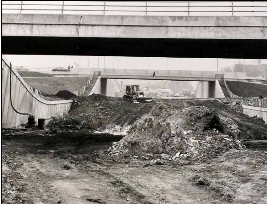
The M32 under construction in the mid-1960s. (Bristol Post)
