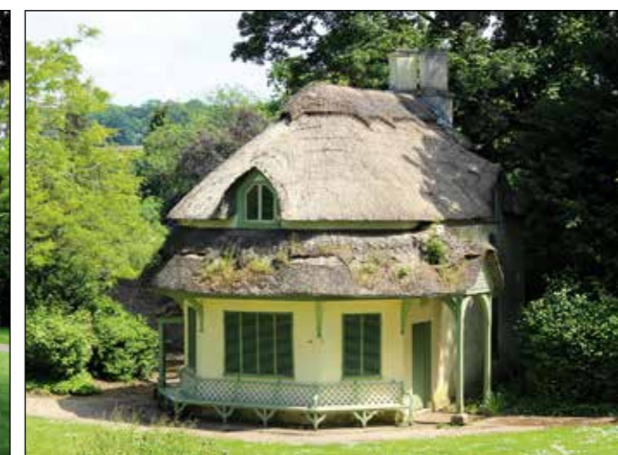
Another unused garden building at Blaise – the Dairy
