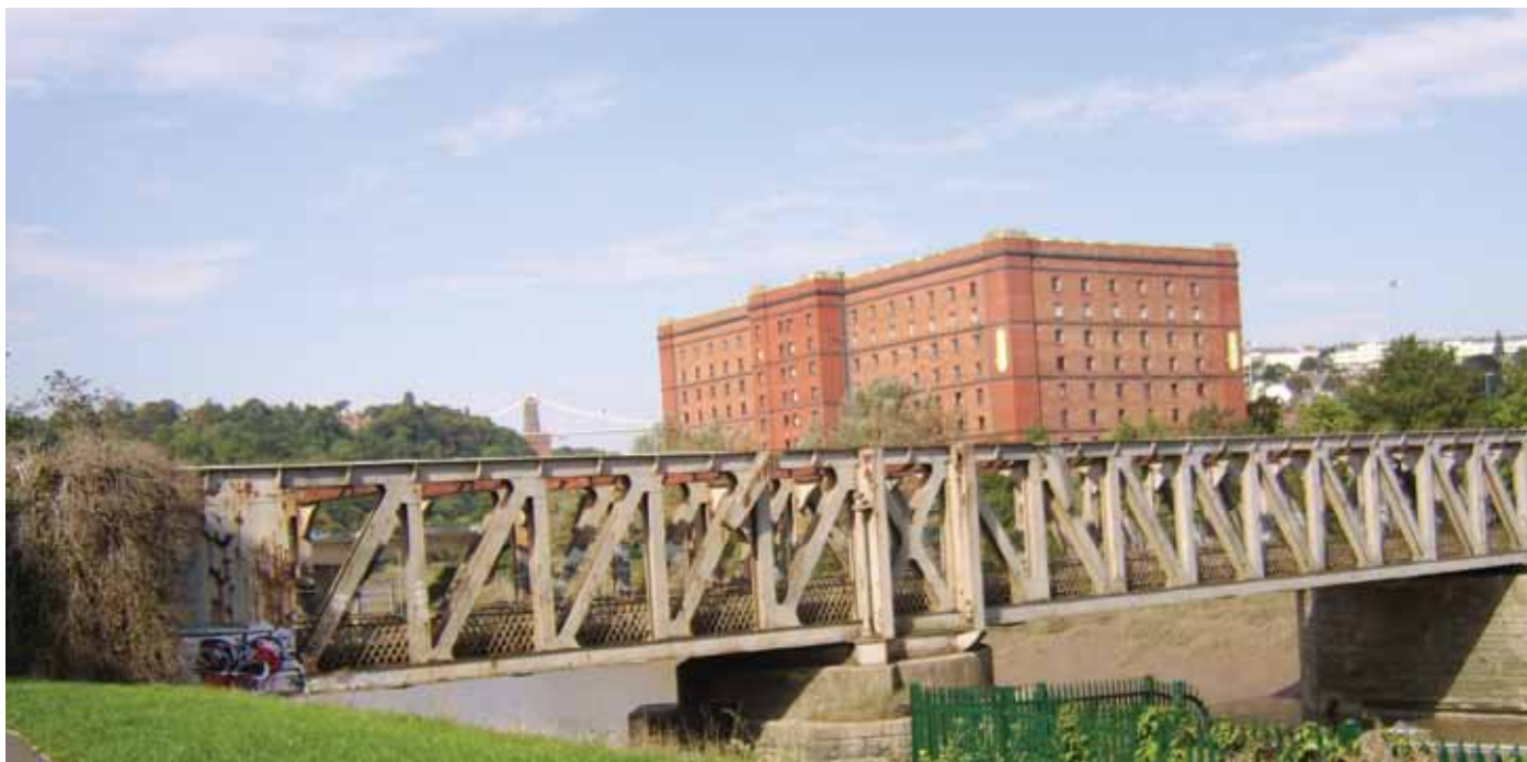
Ashton Avenue Bridge, (Festival Way) - part of the MetroBus, BRT route
