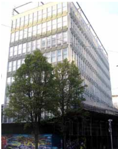
The existing New Bridewell site
