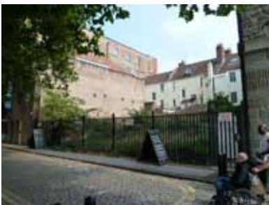
NARROW QUAY "On what must be one of Bristol's photogenic sites, near the Arnolfini, this wilderness cries out to be used properly"
