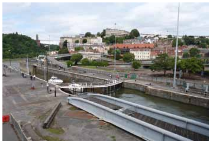
Cumberland Piazza in context of entrance locks and gorge
