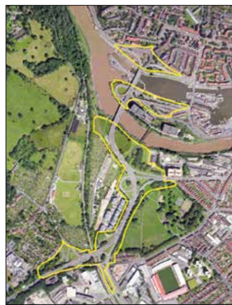
Extent of Scheme, 2012 aerial view.
