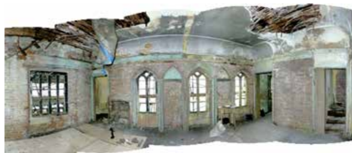
Upper room before work began Ashley-Davies
