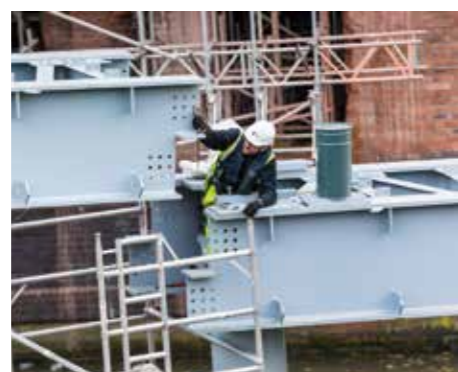
The installation of Finzels bridge.
