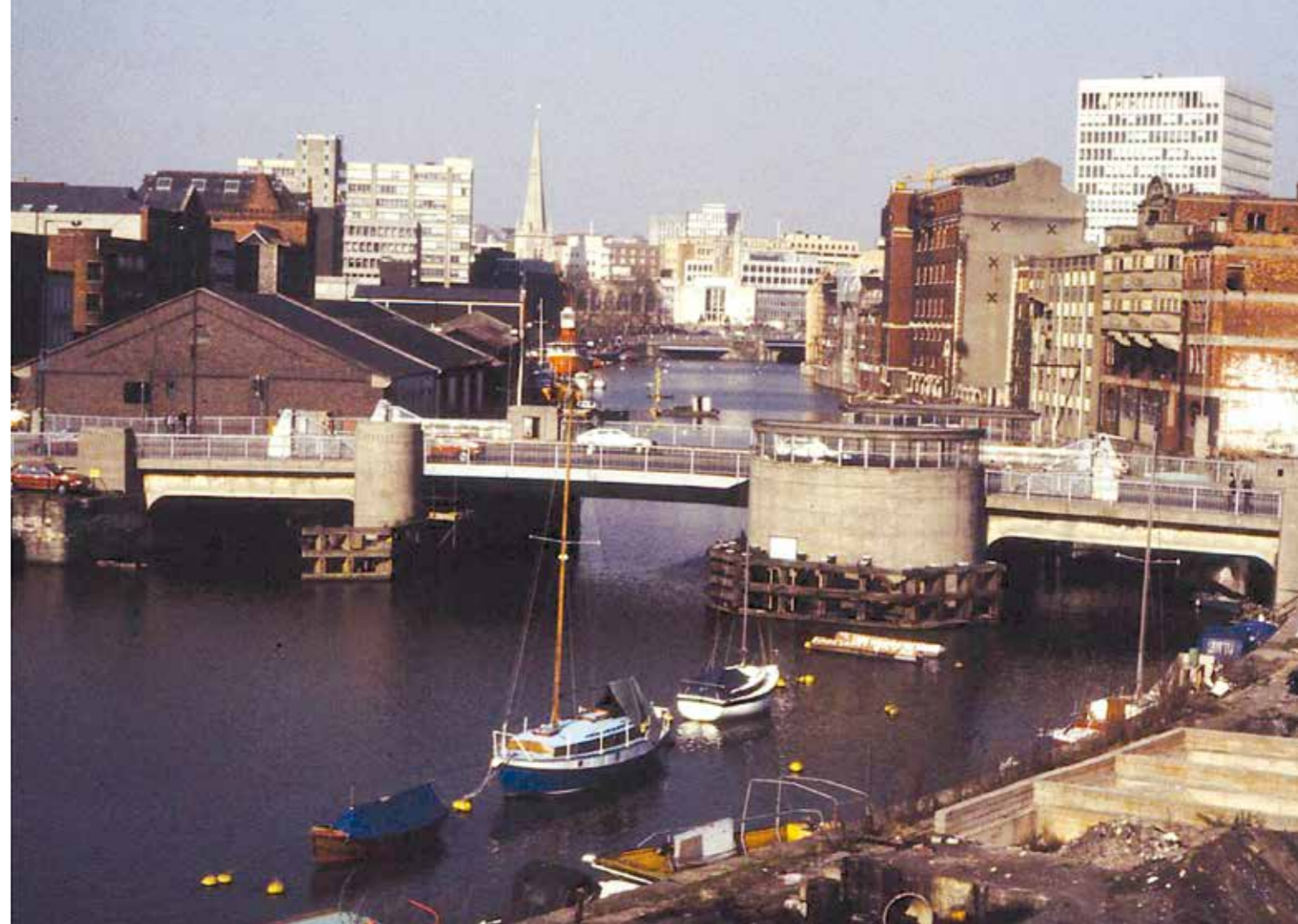
Planners and architects failed to understand the significance of the ancient heritage, street pattern and buildings at the spiritual heart of Bristol.
